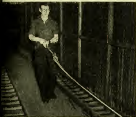
...ing the tubing in the tunnel. Note cooling ladders
